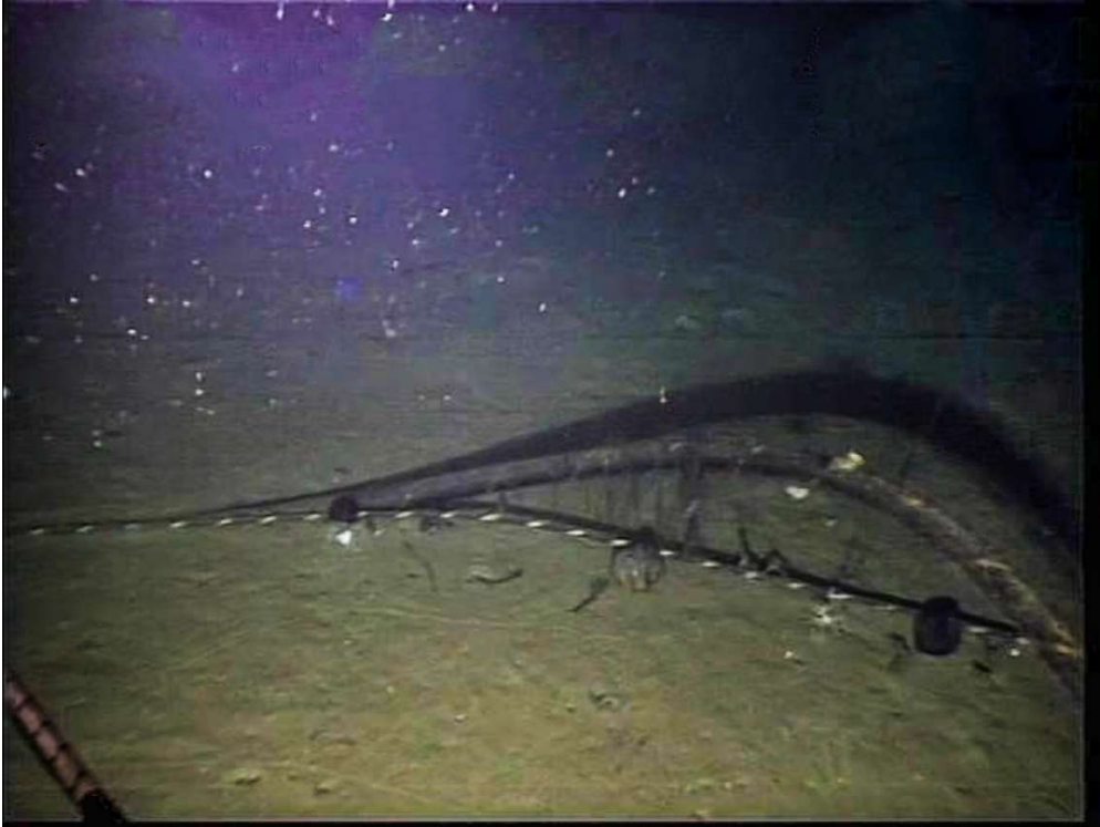
Photos from the initial inspection show the fiber cable damage as well as fiber separating from the power cable.
